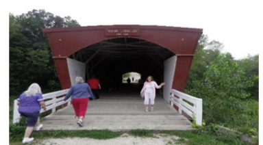
Holliwell Bridge – built 1880
