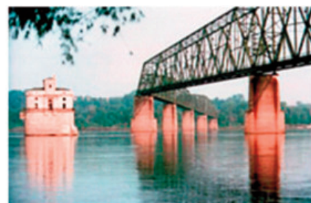
Chain of Rocks Bridge
