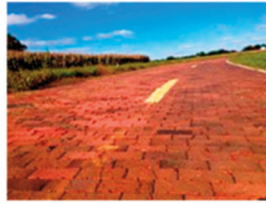
Brick portion of IL 4 north of Auburn
